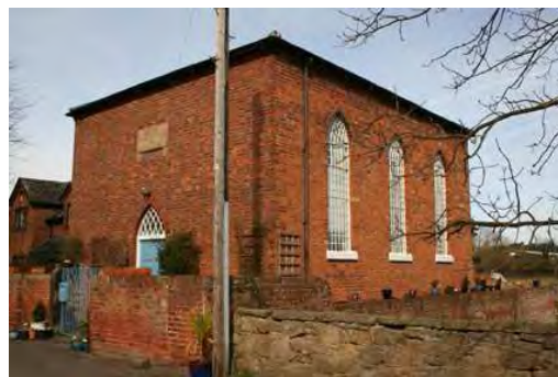
The brick-built Methodist Chapel of 1839
