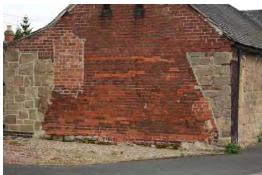
Outbuilding at Walnut Farm
