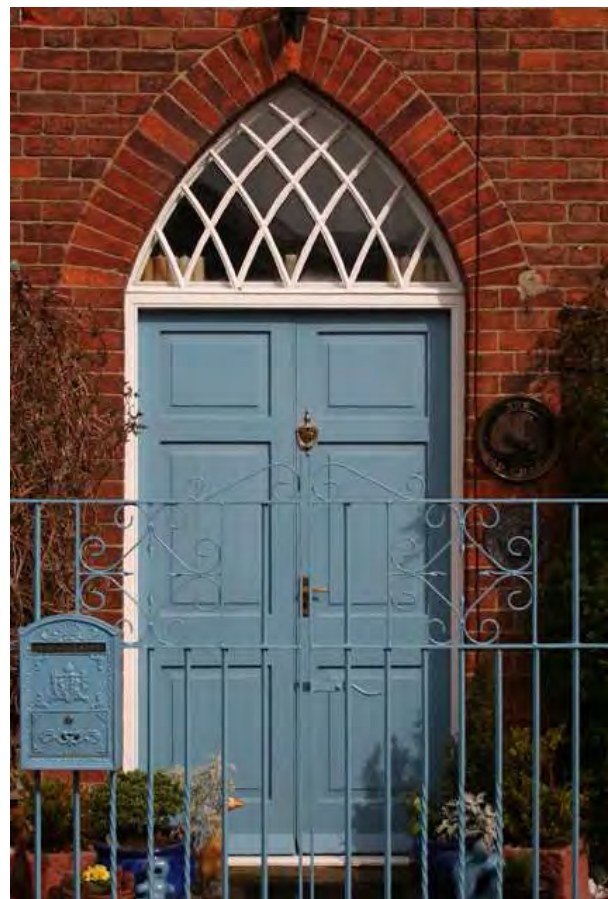
Left - 4-panel door with heavy, applied bolection mouldings at Ivy House, Church Lane.
